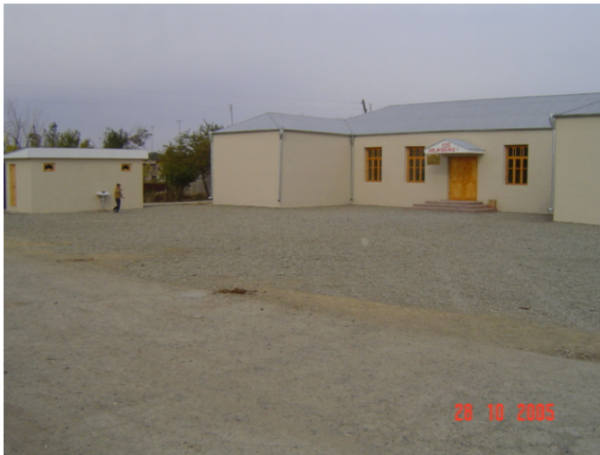
School building and toilet after the completion
